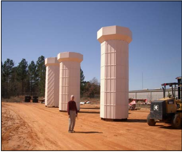
Sections ready for pre-fit
