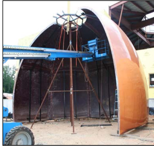
Leaves are loosely placed around an assembly pole (factory supplied on larger domes)
