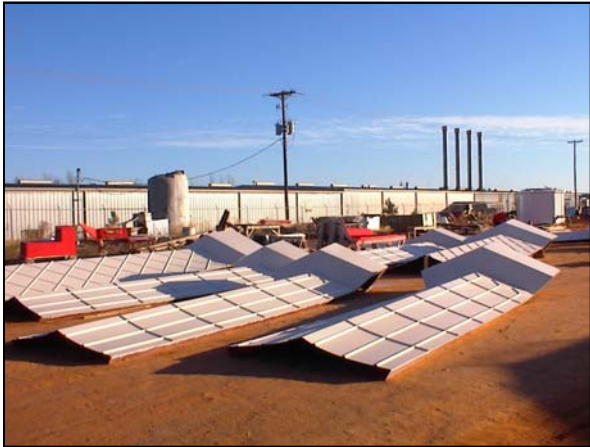
FRP parts ready for assembly
