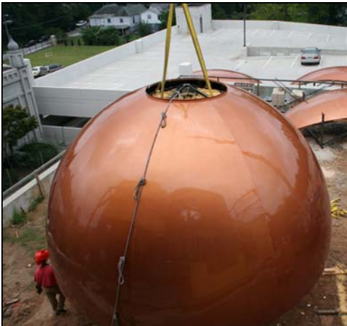
Rigged for lifting
