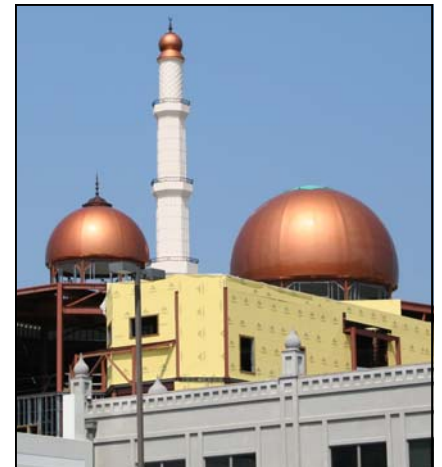
Dome top elements are generally installed via a socket assembly in the top of the dome.
