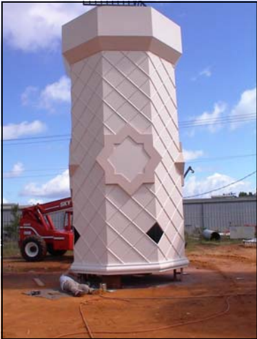
Final assembly (Open panel for light fixture)
