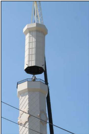
Lift and Install
